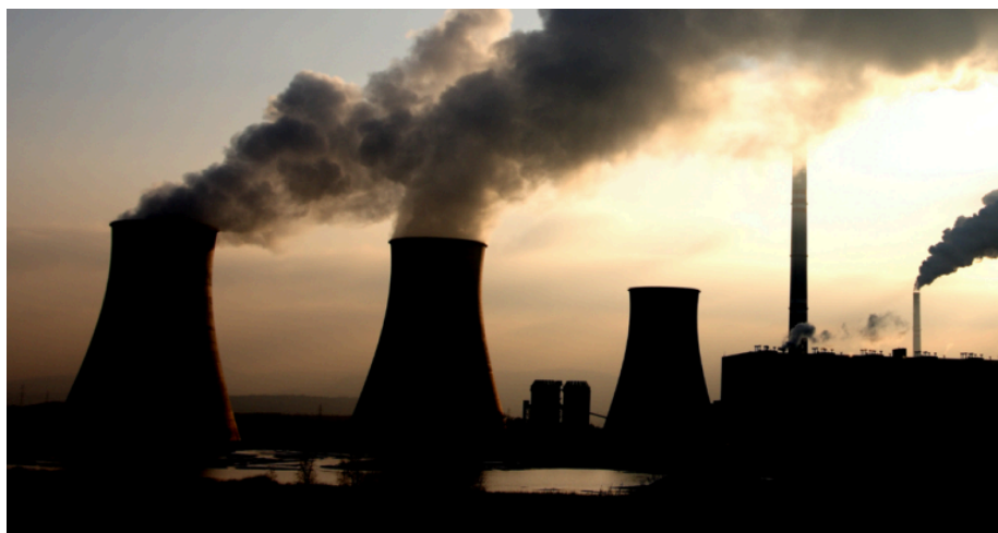
Coal power plant. INQUIRER STOCK PHOTO
