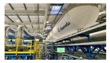
The suspended container can hold around half a tonne of CO2
