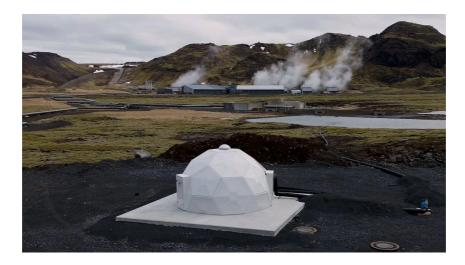
CO2-laden water is pumped underground where it turns to rock
