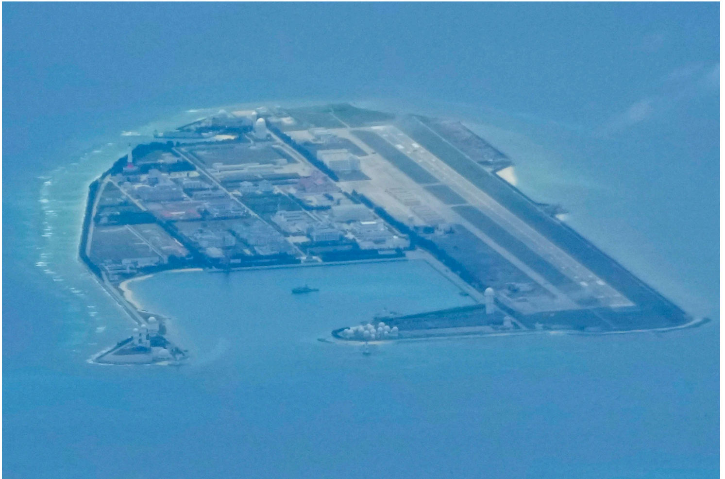
Chinese structures and buildings are seen on a man-made island at Mischief Reef in the Spratly Islands, South China Sea, in 2022. Photo: AP
