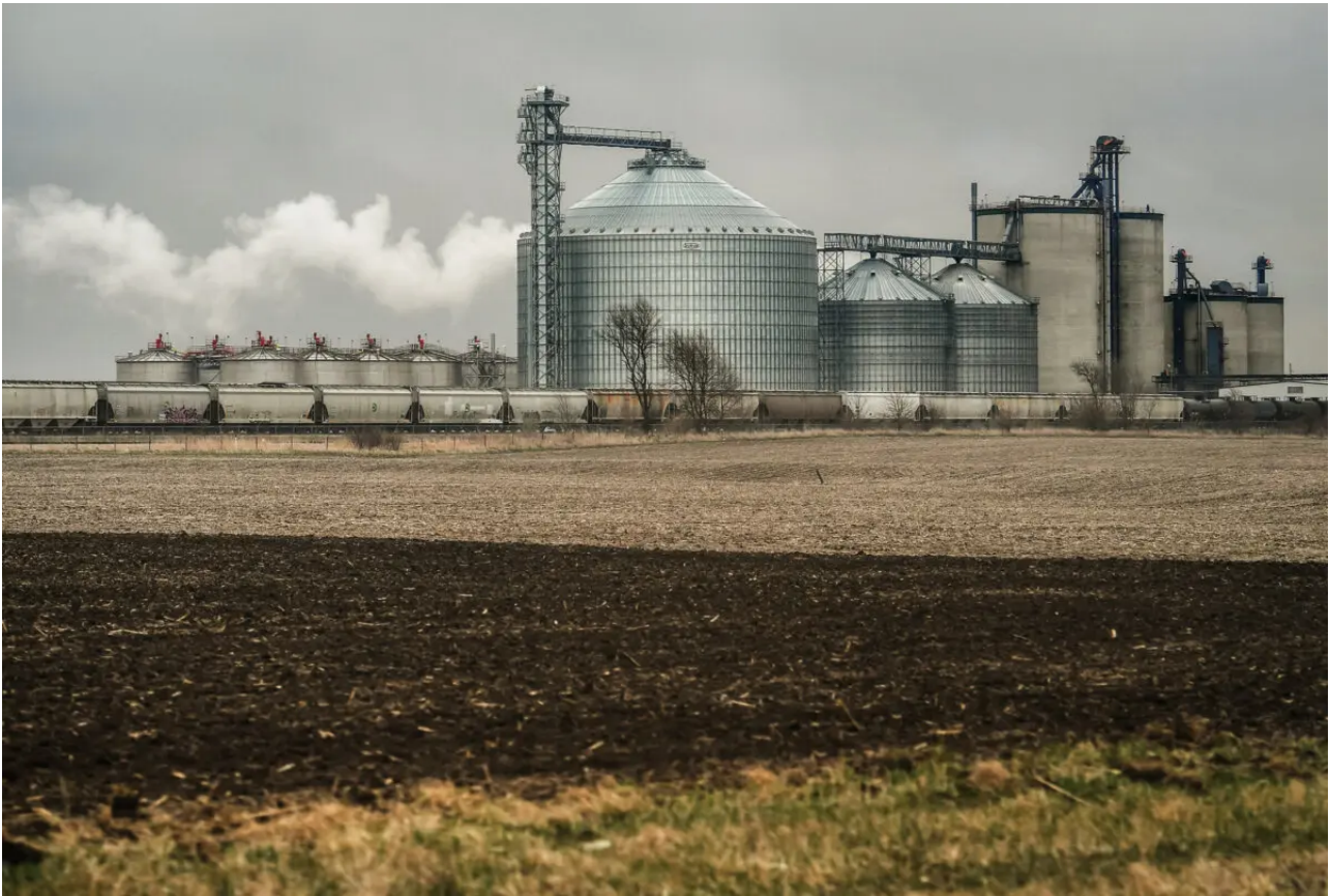
The POET Bioprocessing, a processing plant that produces ethanol, in Menlo, Iowa, on April 12, 2022. (Mandel Ngan/AFP via Getty Images)
